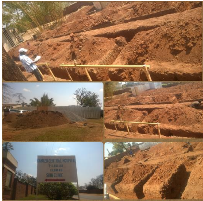
Pictures of the KCH OSC under construction
